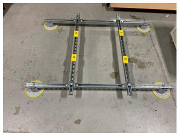
REMOVE HARDWARE AND PLACE ON EQUIPMENT SUPPORT RAIL, SECURE WITH SOCKET
