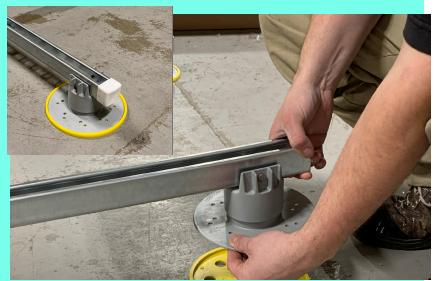
PLACE UNIT USING INCLUDED HARDWARE AND ANTI-VIBRATION PADS IF REQUESTED, OR HARDWARE OF YOUR CHOOSING. ADJUST HEIGHT AND WIDTH AS NECESSARY
