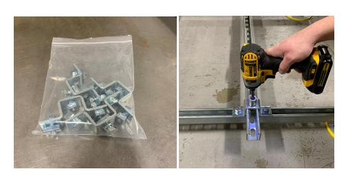
TURN BASE OF STRUT KNUCKLEHEAD UP TO 1" FOR ANY REQUIRED LEVELING. PLACE KNUCKLEPADS UNDER BASE IF INCLUDED INSTALL VINYL END CAPS
