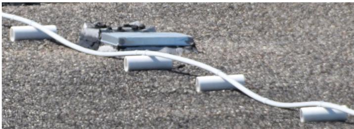
**PICTURE 3:** Inappropriately supported PVC pipe
