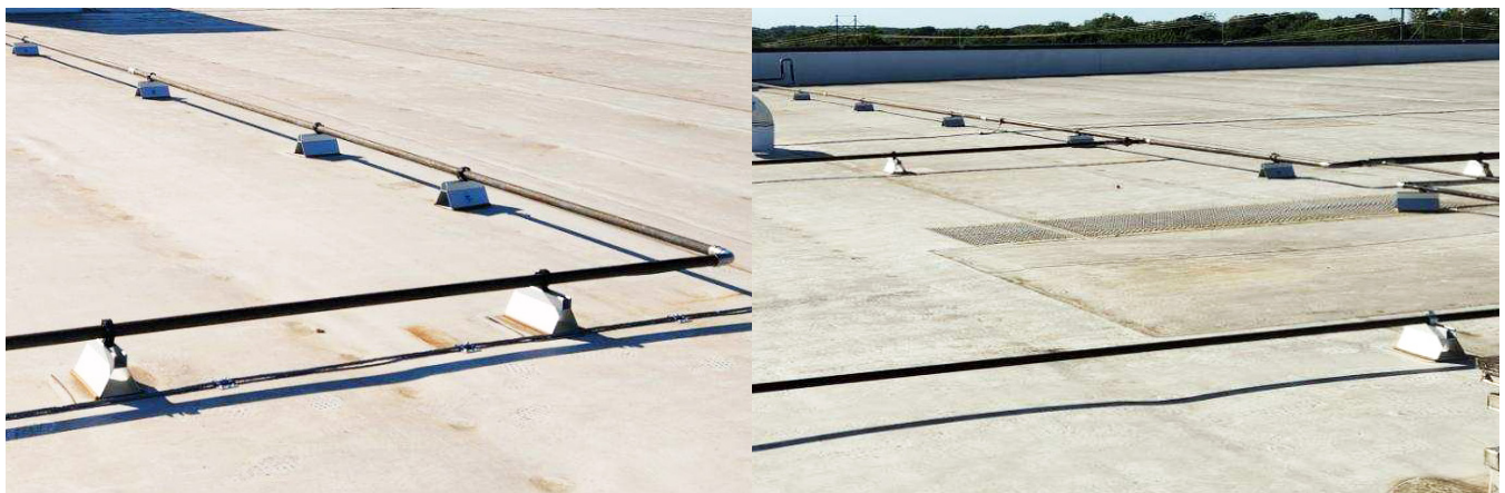
MetalHeads with integrated slipsheets support a lines on a rooftop. The photo on the left shows MetalHeads and Snap-N-Strut clamps. The right-hand photo shows MetalHeads using pipe clamps provided by others.
