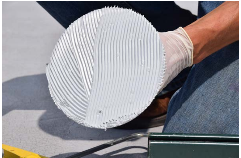
Green Link Adhesive/Sealant application. In this instance the KnuckleHead will be bonded with adhesive to a fully adhered membrane.
