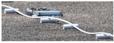
PICTURE 3: Inappropriately supported PVC pipe
